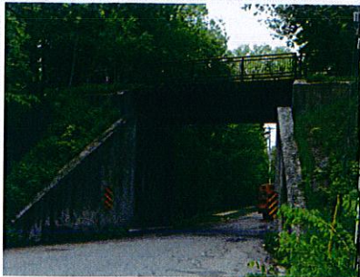
➤ Emily Street Underpass
