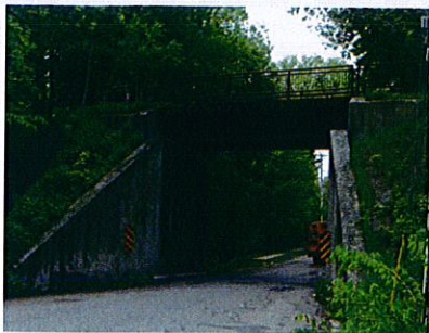
➤ Emily Street Underpass
