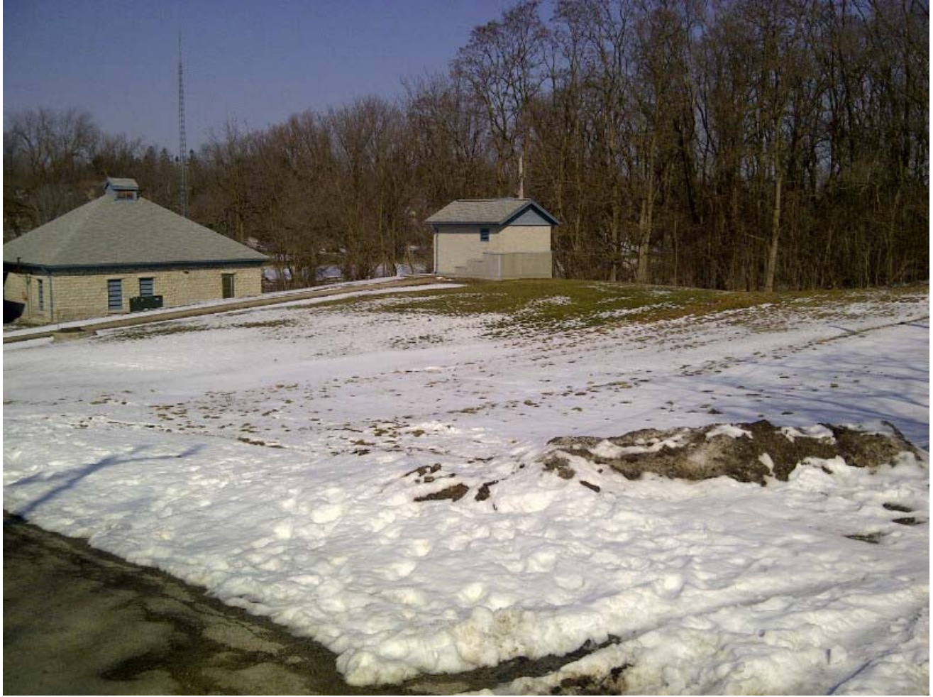
Well Site 1 – looking east from St. George St. North, showing existing well house and water treatment building.
