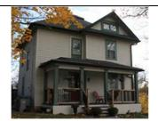
This two-storey house, built in 1909, is a good example of utilitarian, box-shaped, balloon-framing house construction, common in St. Marys from approximately 1890 into the 1930s.
