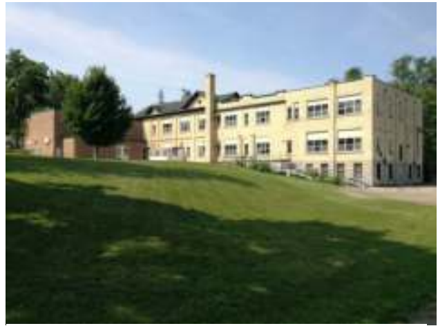
The former Arthur Meighan Public School, as viewed from Wellington Street
